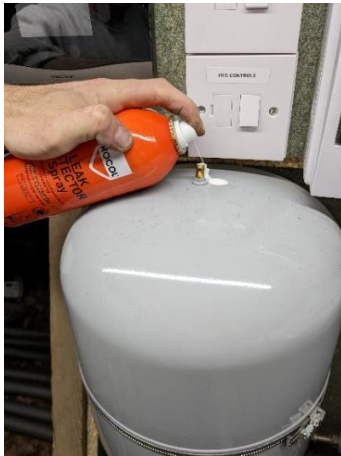
Pic.7 – Testing Schrader valve
