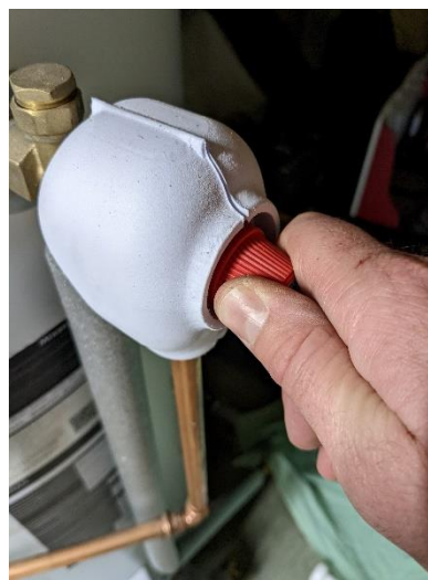
Pic.15 – Check exp. Vessel precharge Pic.16 – Check T&PR Valve
