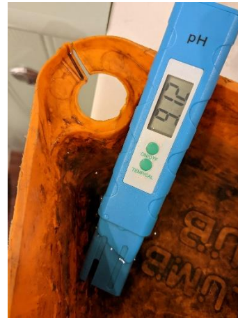
Pic.9 – Heating system pH test
