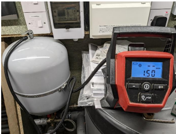
Pic.5 – Exp. Vessel testing
