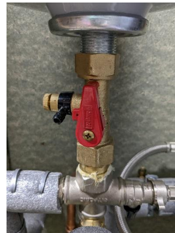
Pic.6 – Exp. Vessel service valve
