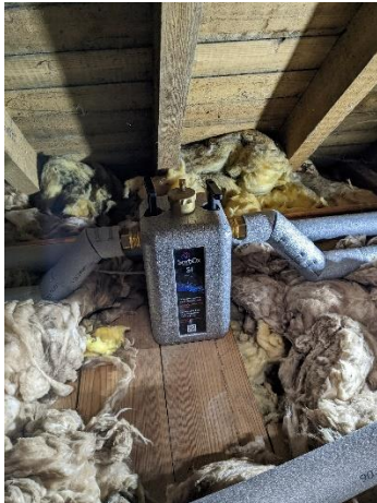
Pic.14 – Sorbox Si anode test
