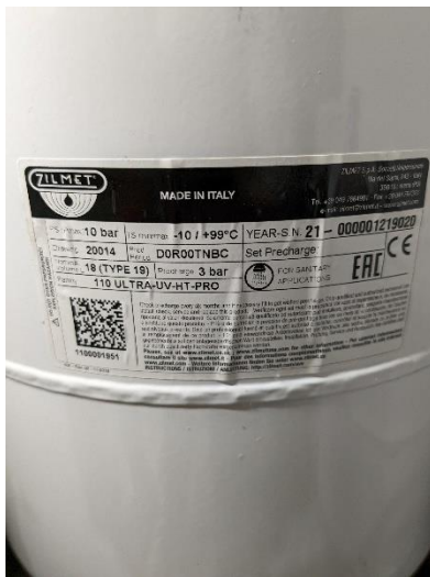
Pic.15 – Check exp. Vessel precharge Pic.16 – Check T&PR Valve
