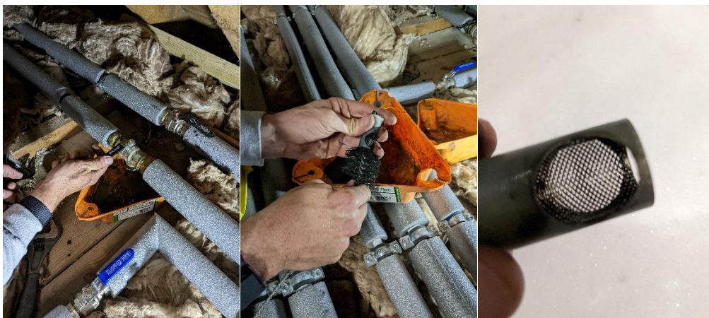
Pic.5 – Cleaning strainer
