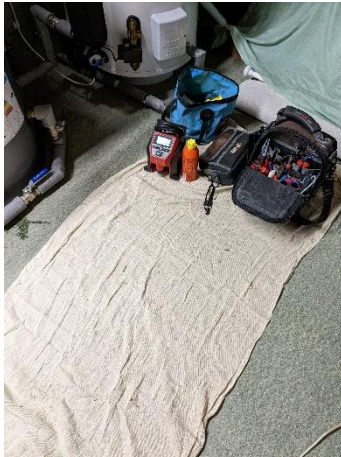
Pic.1 – Example work area with dust sheet
